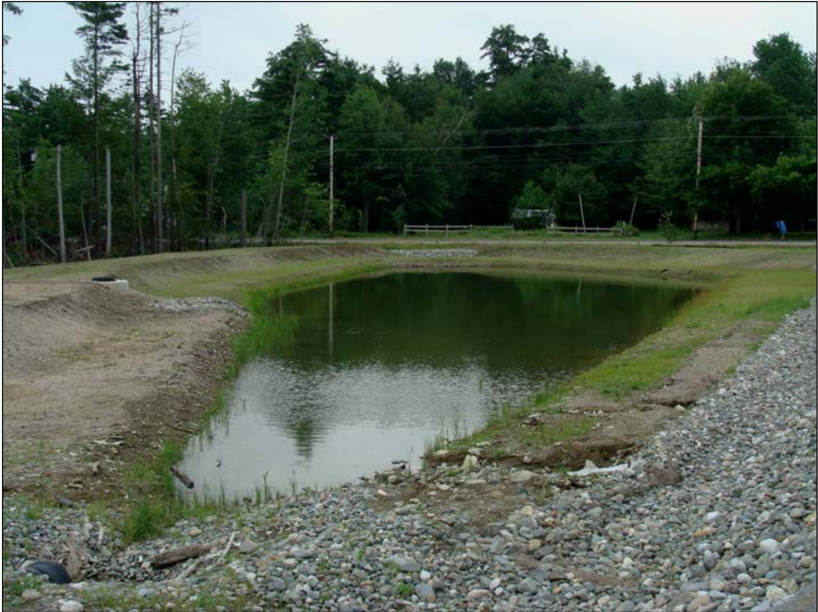
Not a vernal pool - retention basin, often permanent and low water quality
